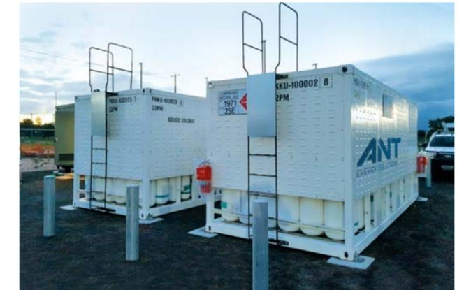
20 ft containers for holding 2.2 MW hrs of electricity equivalent
